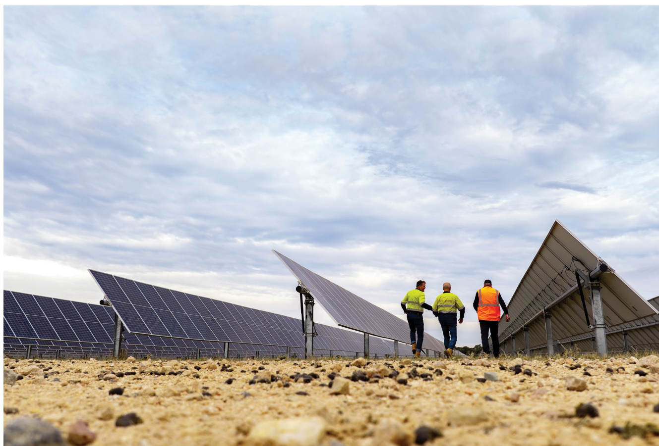
Darlington Point Solar Farm, NSW, Australia.
