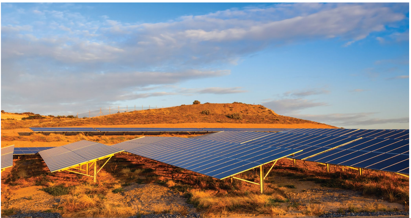
Solar farm, South Australia, Australia.
