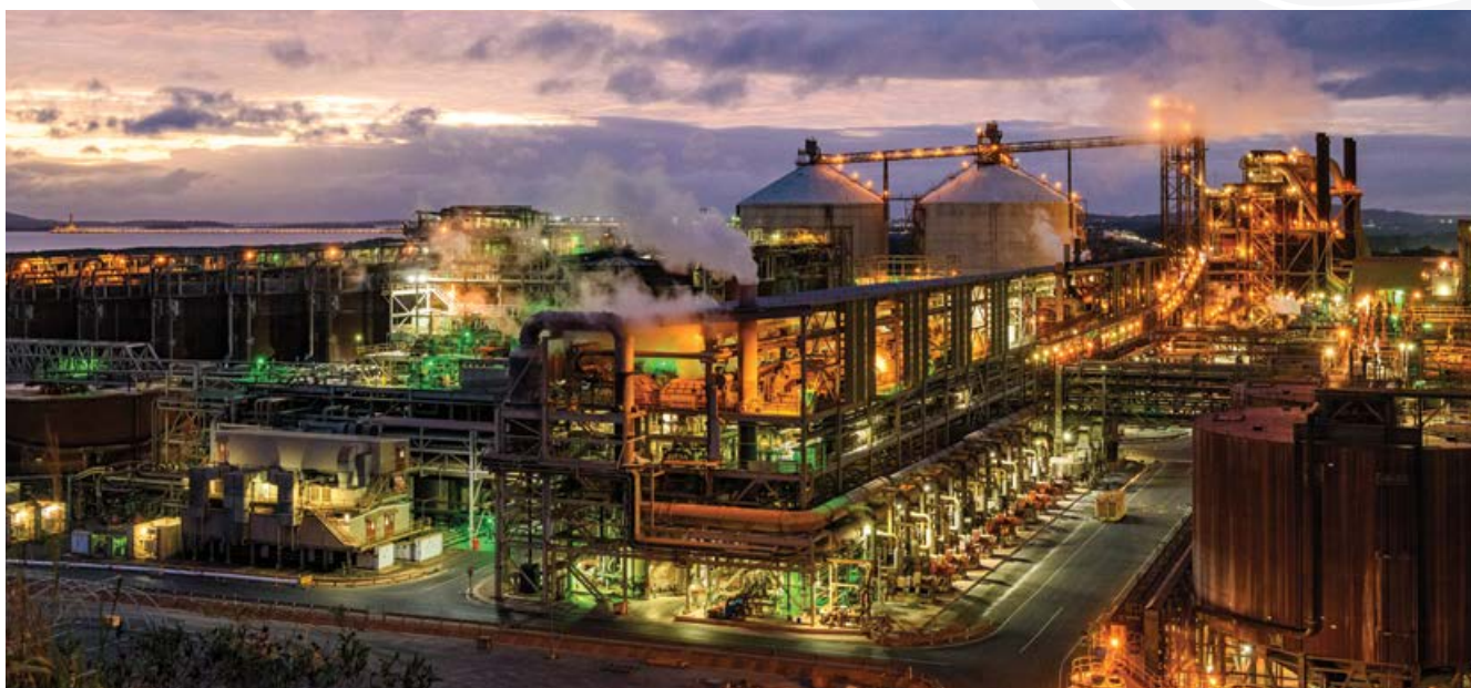
Rio Tinto Yarwun Alumina Refinery, Gladstone, Queensland, Australia. Credit: Rio Tinto.
