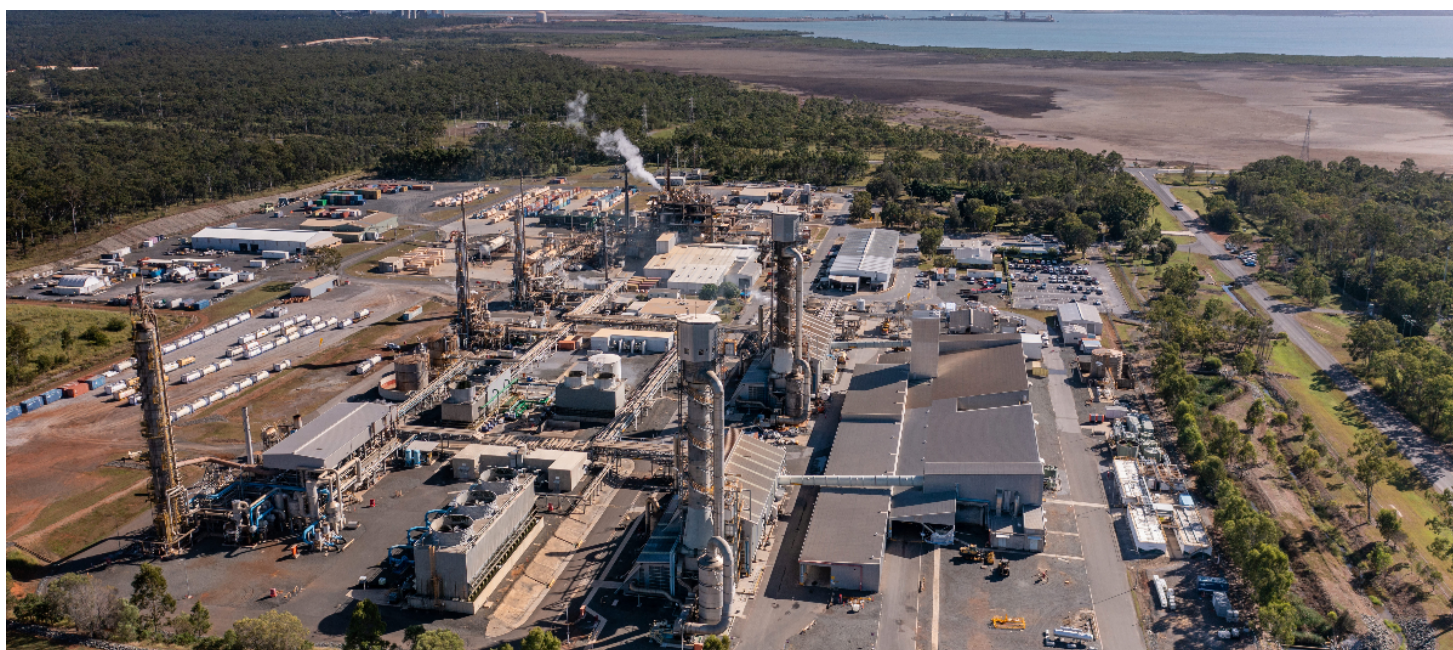
Orica Yarwun Manufacturing Facility
