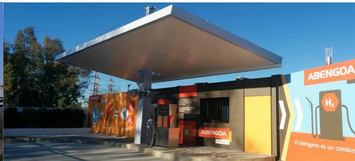
Torrecuéllar HRS with onsite production of 30 Nm 3 /h
